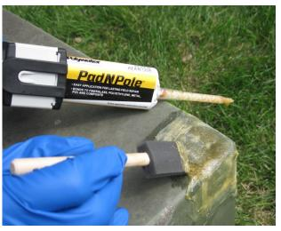
Fiberglass cloth saturated with the high-strength, two-part resin makes the permanent PowerPatch<sup>®</sup> Pad N Pole<sup>™</sup> Repair.
