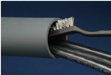
Clean duct with wire brush, solvent wipe.
