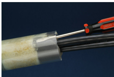
Use screwdriver to check for voids
