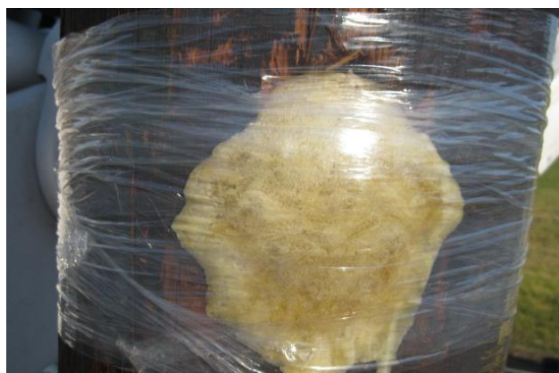
Woodpecker damage repaired with UPR™ Pole Repair
