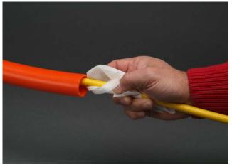
Polywater® FTTx Spray Lubricant remains effective with very thin, molecular-level films, so it continues to lubricate even when it cannot be detected.
