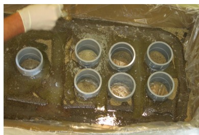
Spread the InstaGrout™ material with stir stick
