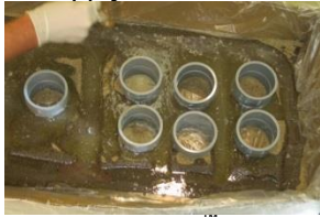
Spread PedFloor™ with stick
