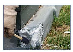
6. Generously apply additional Pad N Pole™ adhesive to the top of the fiberglass cloth (including the cloth over the hole) and smooth with the brush until the cloth is fully saturated. Brush the Pad N Pole™ adhesive ½ inch (1.3 cm) past the edges of the cloth, feathering the resin and ensuring that the edges of the cloth are well adhered to the surface. Pad N Pole™ adhesive will set in about 30 minutes and reach full strength in about 12 hours.
