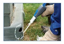
4. Cut the fiberglass cloth to overlap the damaged area by approximately 1 inch (2.5 cm). Generously apply the two-part Pad N Pole™ adhesive to the cleaned surface around the damaged area.
