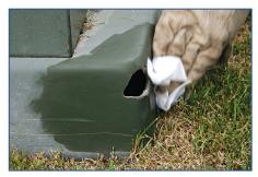
Clean and dry the abraded area with the included cleaner to remove contaminants. Proper adhesion of repair requires a clean surface.
