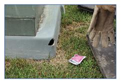
Abrade the area to be repaired approximately 1½ inches (3.8 cm) around the damage using the abrasive cloth included in the kit.
