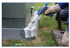
5. Lay the fiberglass fabric over the damaged area, pressing the edges into the Pad N Pole™ adhesive. Smooth and press down with the foam brush. The patch will cling to the adhesive covered area and quickly saturate with the Pad N Pole™ adhesive.
