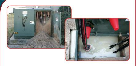
Polywater® InstaGrout™ helps prevent outages and service disruptions by creating a resilient and impermeable barrier. InstaGrout™ is an excellent electrical reliability sealant that keeps out moisture and stops rodents, snakes, spiders, wasps, and fire ants from burrowing up through earthen gaps into the pad enclosure.
