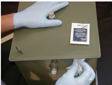
Clean area with cleaning wipe before applying PowerPatch ® Putty
