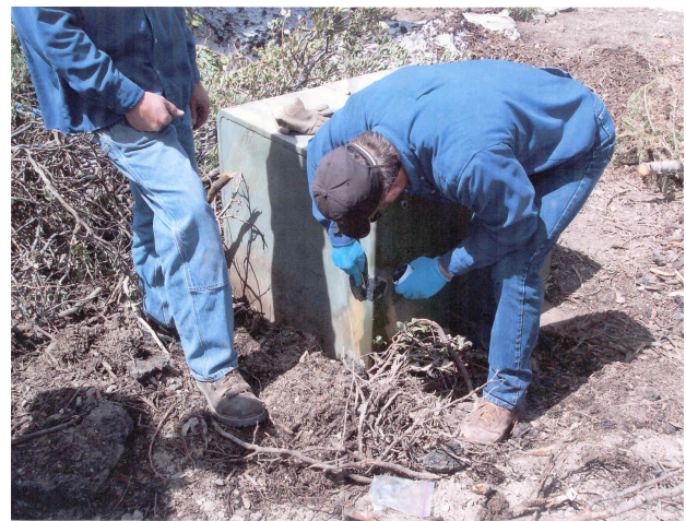
PowerPatch ® being applied to transformer.
