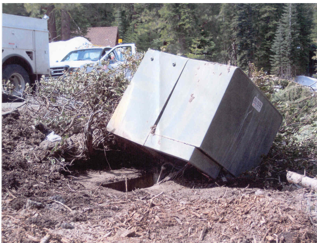
Transformer hit by snow plow.
