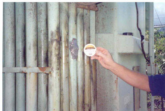
PowerPatch ™ repair of leak.
