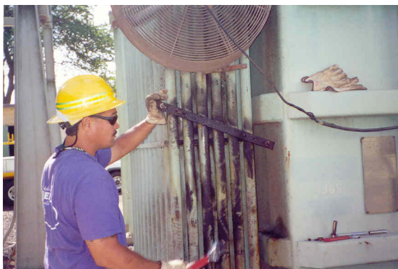
Bracket being removed to locate leak.
