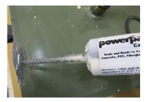
Apply PowerPatch<sup>®</sup> Sealant over putty patch or leak area
